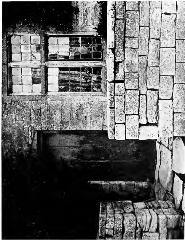
DETAIL OF HOUSE AT BIERLY The door step is well worn by years of use
